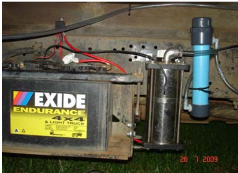
Relay installed on the left
